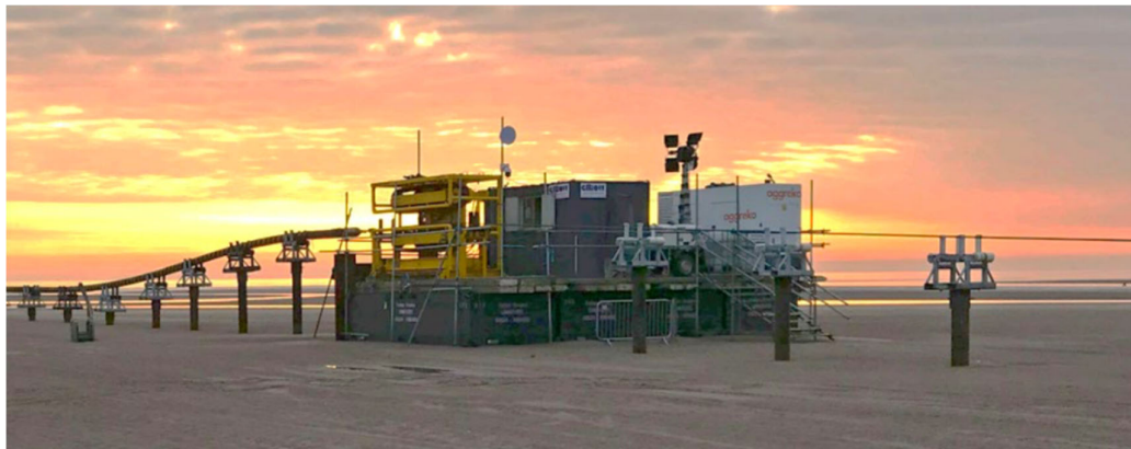
Plate 3.6: Example roller boxes and intermediate pulling platform installation (image courtesy of Boskalis)
