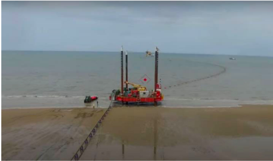
Plate 3.7: Example intermediate pulling platform barge
