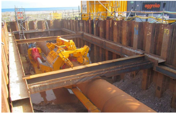
Plate 3.4: Direct pipe thruster equipment at the landfall compound
